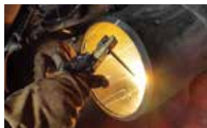
Shielded metal arc welding
