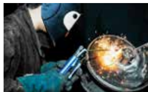
Arc welding with tubular electrodes
