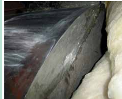
Rebuilt furnace support roller
