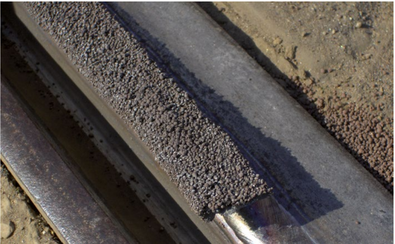
BF 4 with tubular wire Ø 4,00 type 18.8.6 L Excellent weld bead appearance, also in rail crossings and bends.
